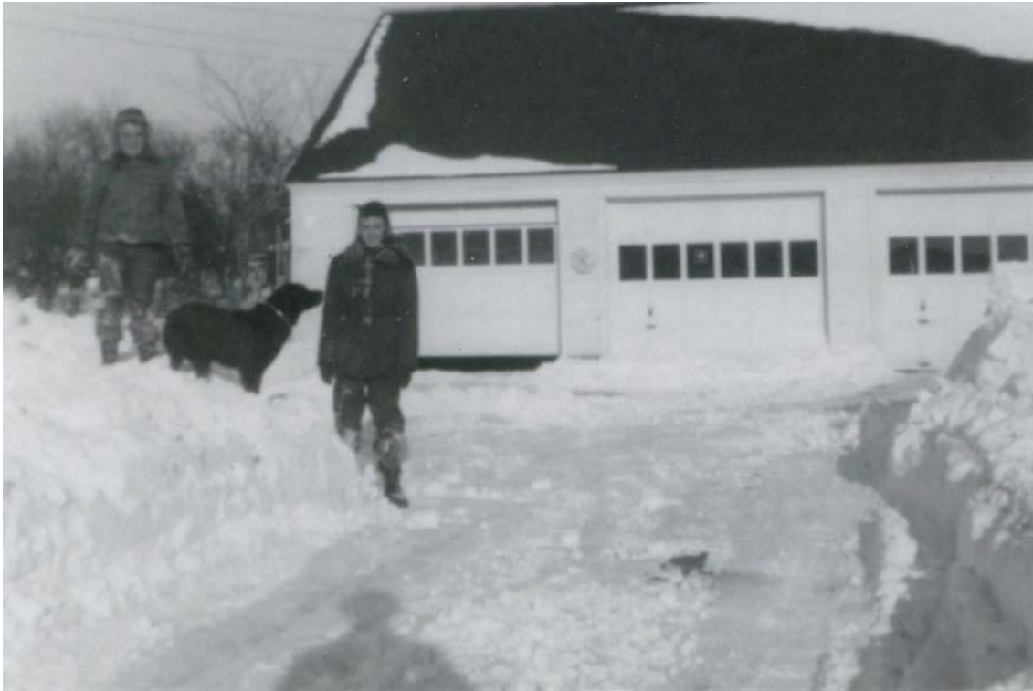
New Garage built in 1950-Jeanette & Leon Westerfeld with “Pooch”.
